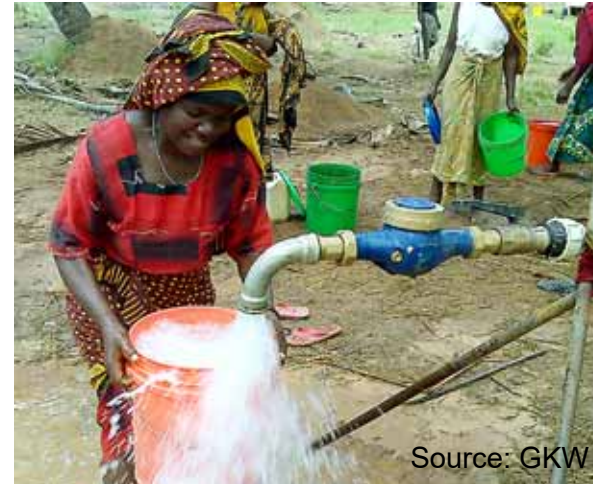
Town supply upgrade, Tanzania
